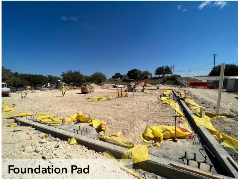
Partial Slab Formed
