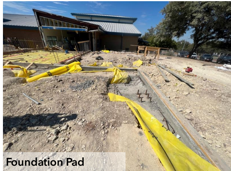
Partial Slab Formed
